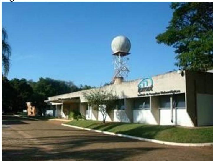
Figura 10 – Fachada IPMET Bauru – Radar Banda-S
