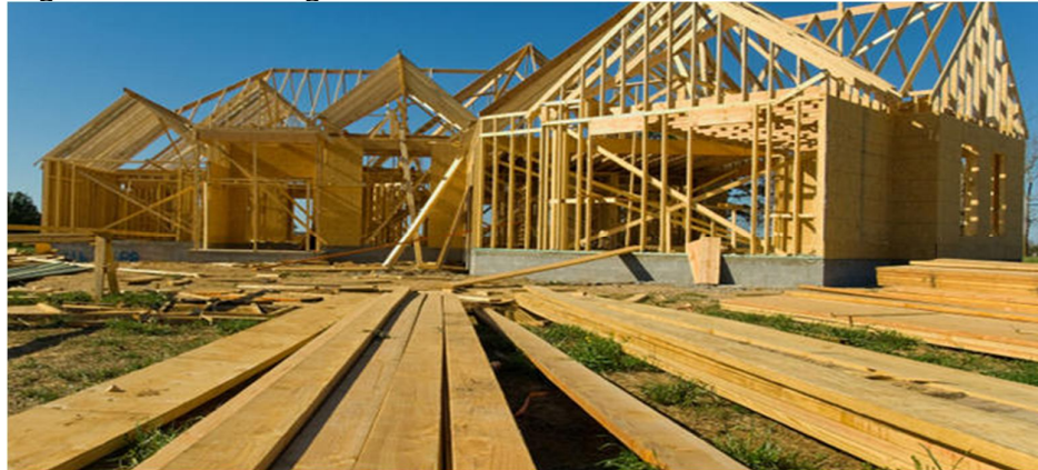
Figura 16 - Wood Light Frame
